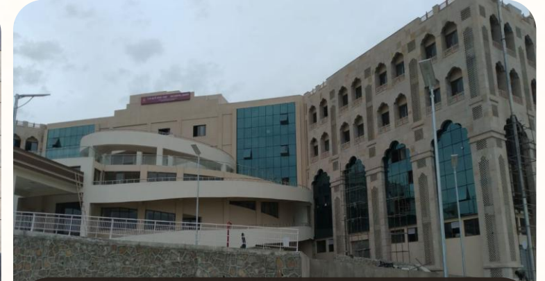
Hospital Project In Udaipur Rajasthan
