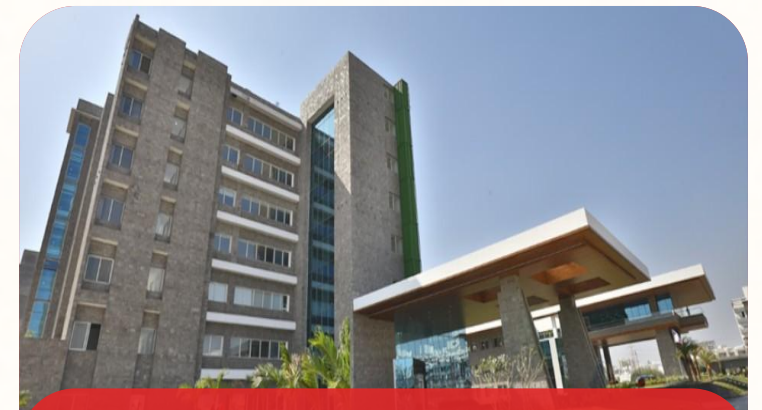
R&D Centre at Vadodara
