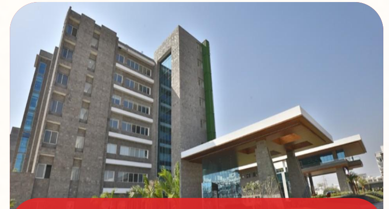
R&D Centre at Vadodara
