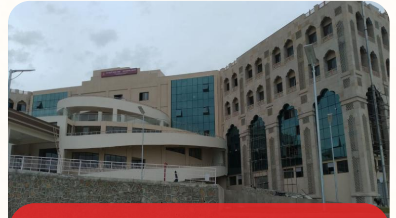
Hospital Project In Udaipur Rajasthan
