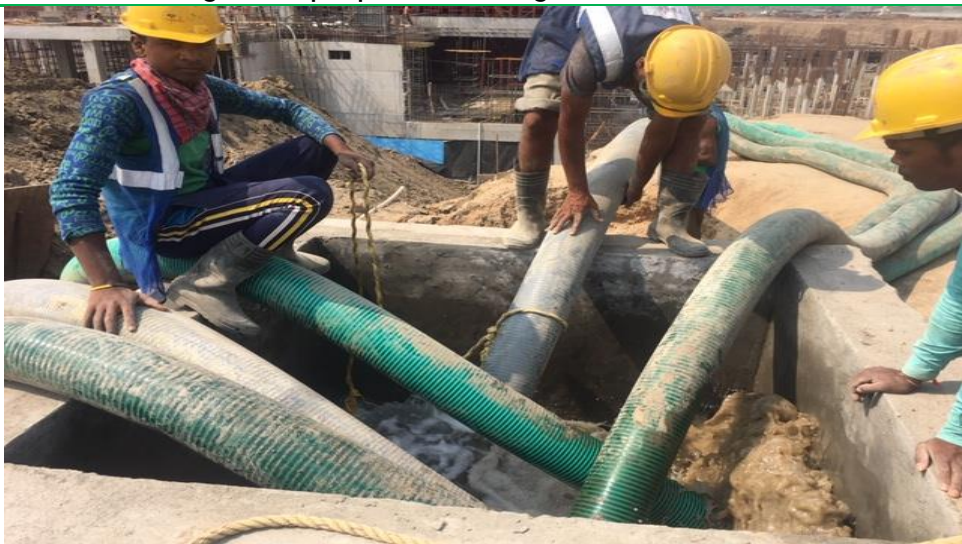
Exhibit 1: PSP using electric pumps for dewatering
