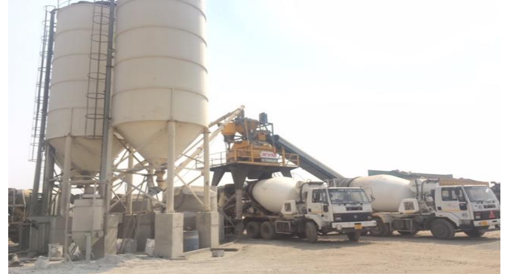
Exhibit 6: Concrete batching plant, cement procured from JK Laxmi and Ultratech
