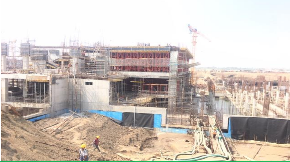
Exhibit 3: Basement, G-1 construction work for all towers progressing smoothly
