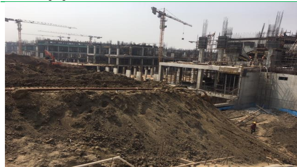
Exhibit 2: Ongoing work at the site
