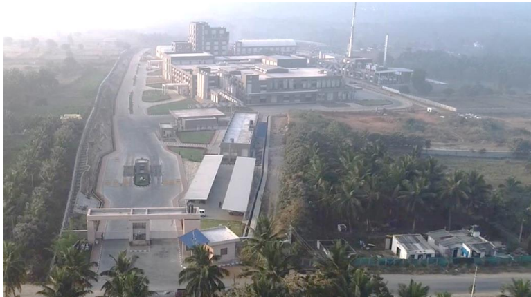
BANGALORE MILK UNION DAIRY PLANT AT KANAKPURA, KARNATAKA
